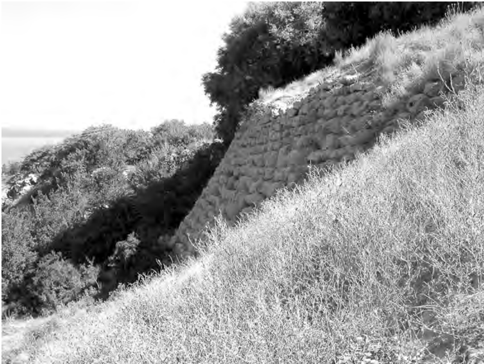
Figure 130 Embankment of Minua canal at Edremit, 8 km south of Van.
