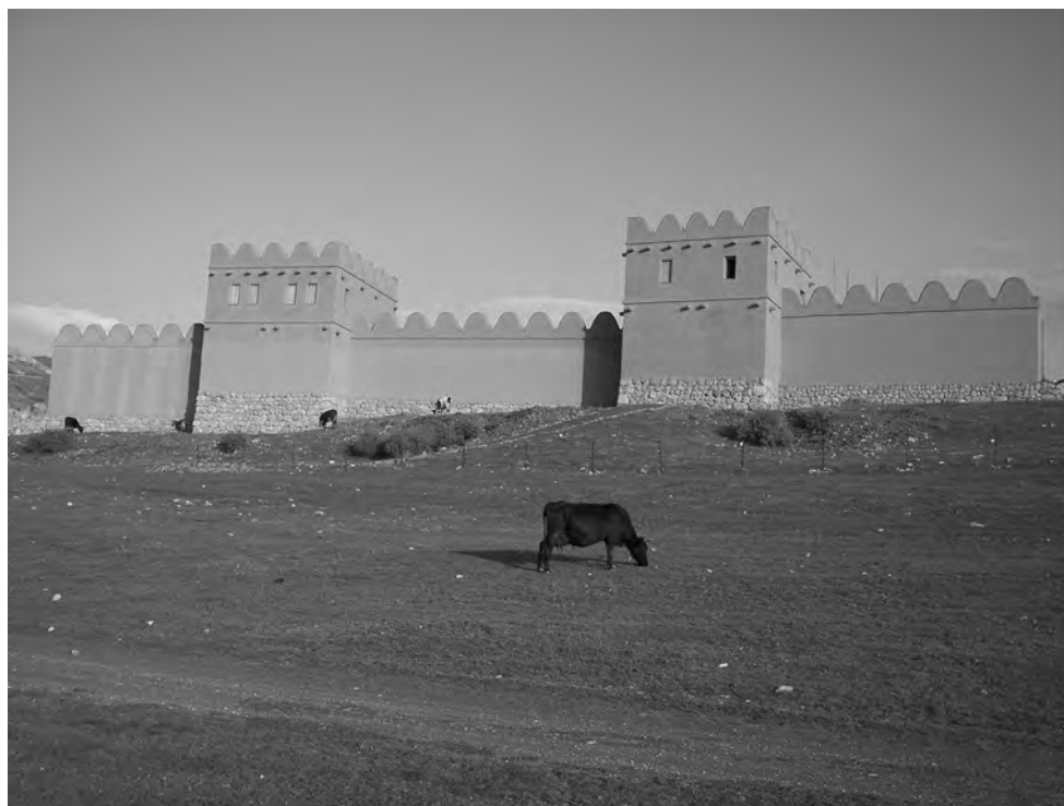
Figure 48 Hattusa, reconstructed wall.
