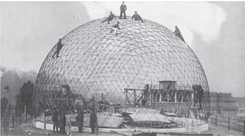
Figure I.2.3 Building an experimental dome at the Carl Zeiss factory. Photograph Popular Mechanics , 1929.
